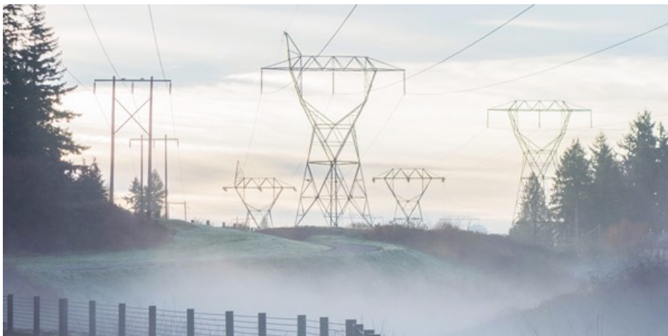
Avangrid transmission lines | UWUA
