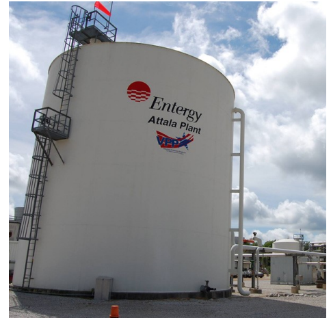
Attala Plant | Entergy
