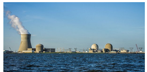
The Salem and Hope Creek nuclear plants, which PSEG CEO Ralph Izzo claims will become unprofitable in about a year.
